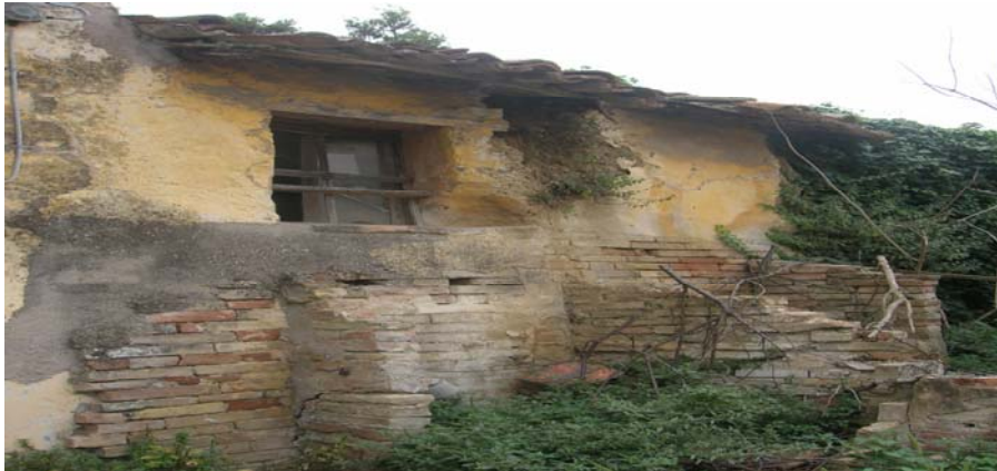
Figure 2. Typical raw-earth cob architecture at “Villa Ficana” in Macerata (Italy). An external masonry staircase is often present to connect the two levels of the house. A masonry support is also visible low on the left.
