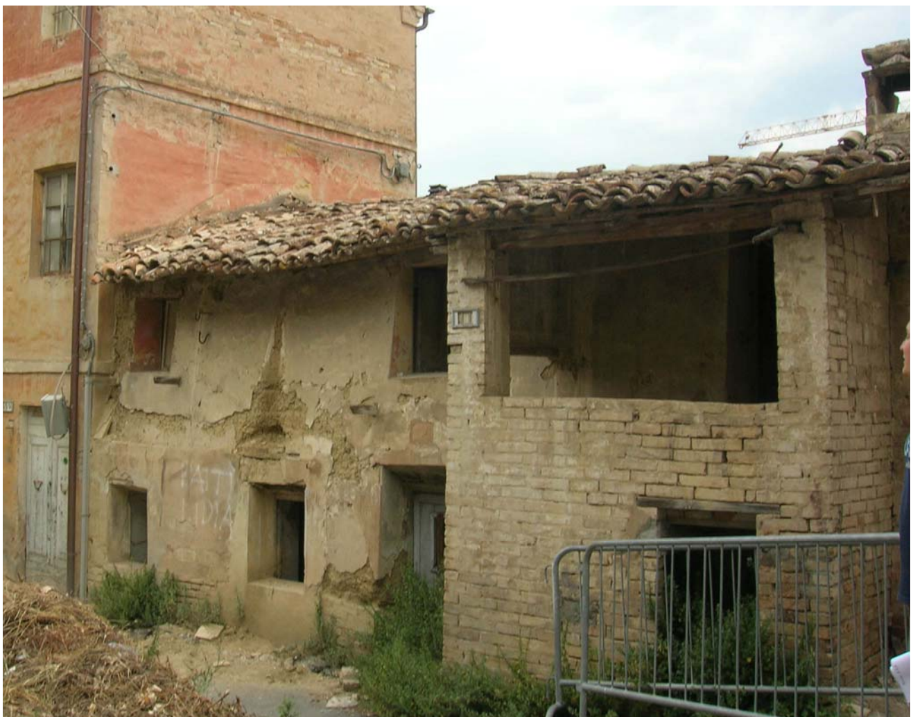
Figure 2. Typical raw-earth cob architecture at “Villa Ficana” in Macerata (Italy). An external masonry staircase is often present to connect the two levels of the house. A masonry support is also visible low on the left.
