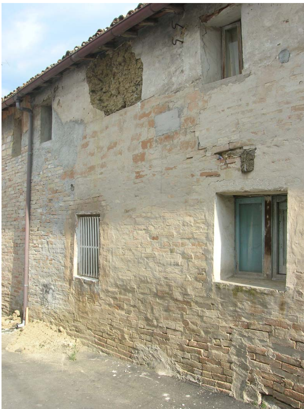
Figure 3. Raw-earth cob walls are often safeguarded by a thick earthen plaster or by a layer of fired bricks.
