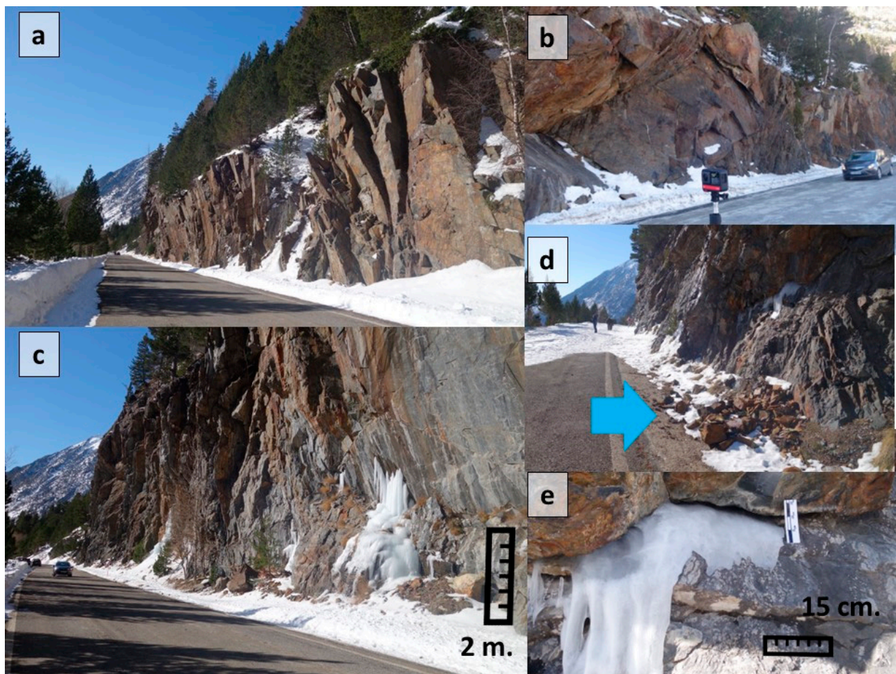
Figure 4. Study site 2: Llanos del Hospital (Benasque, Pyrenees) cross-country ski resort and road to the French border. Temperature during the field trip day (maximum) +4 °C, night −12 °C. (a) Toppling problems at slope 6; (b) wedge failure at slope 9; (c) toppling and ice falls at slope 8; (d) fallen blocks; (e) frozen joints and ice cracking.
