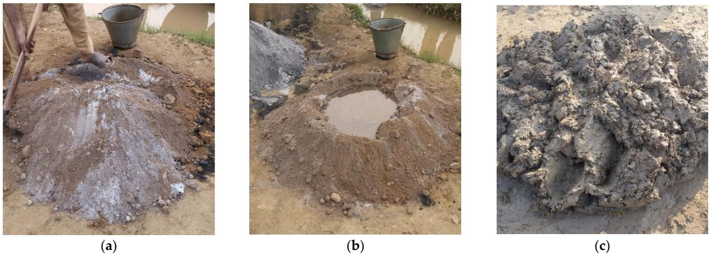
**Figure 2.** Mixing of materials used for brick manufacturing. (a) Dry mixing of ingredients; (b) Adding water to the dry mixture; (c) Wet mixing of ingredients.
