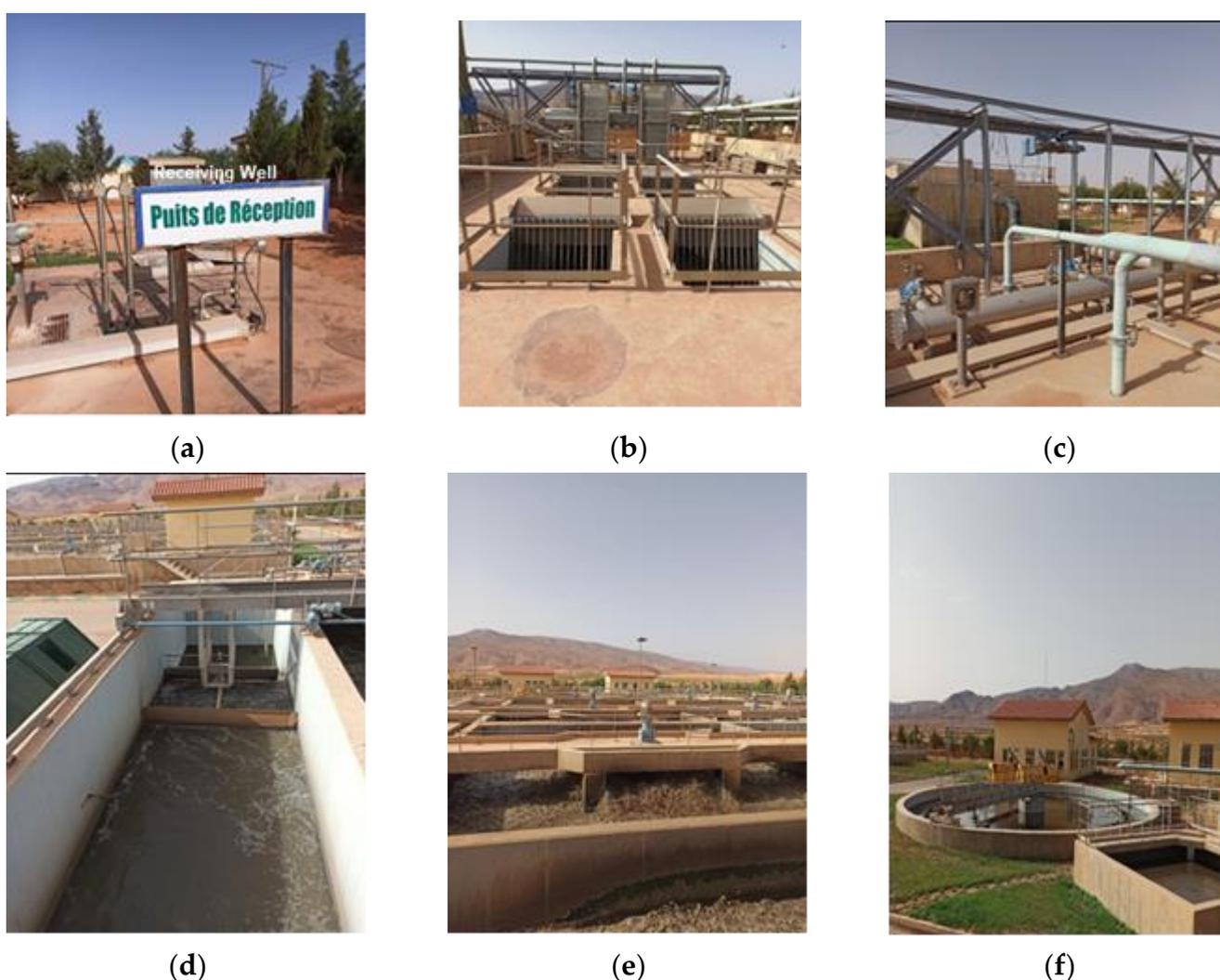
**Figure 2.** Treatment Processes of the WWTP of Ain Sefra ((a): receiving well; (b): screening; (c): pumping station; (d): sand and oil removal; (e): aeration tank; (f): clarification basin).
