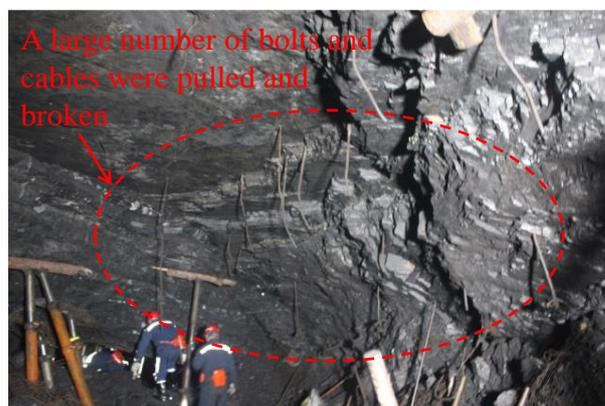
Figure 3. Photo of the anchor bolt (cable) breaking.
