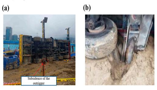
**Figure 5.** Overturning accident from mobile crane. (a) Mobile crane overturning accident and (b) outriggers more than 2 m into the ground.
