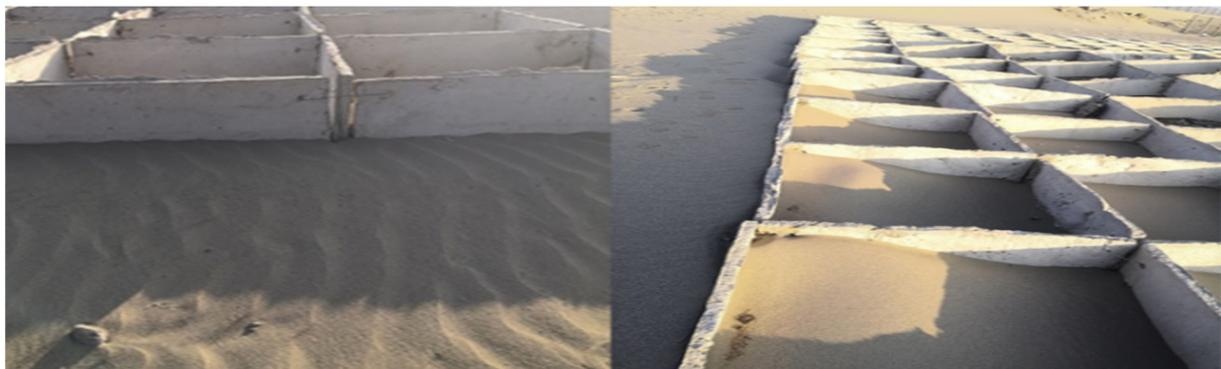
Figure 24. Sand-fixing effect of the checkerboard sand barrier.
