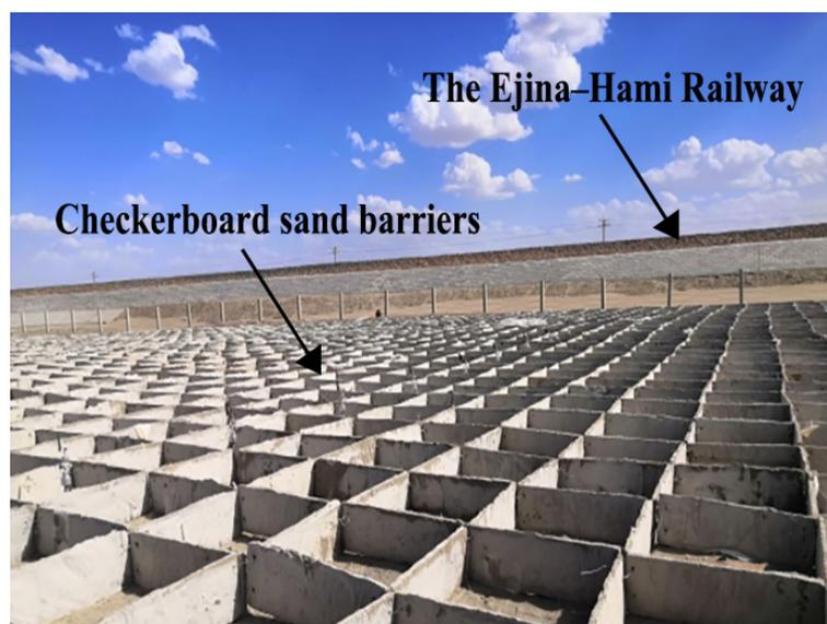
**Figure 21.** Checkerboard sand barriers along the Ejina-Hami railway line.
