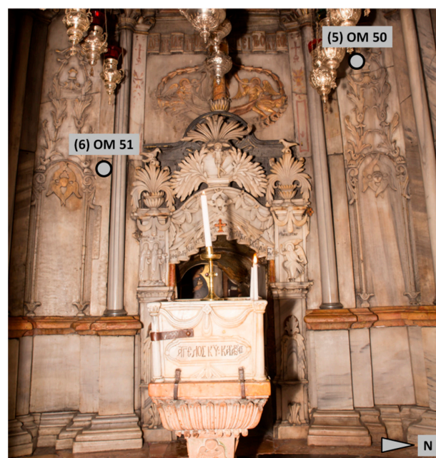
Figure 9. Description of sampling areas of marble samples (5) OM50 and (6) OM51 in the Chapel of the Angel; At the right hand side-northern to the Tomb Chamber entrance, the sampling area of sample (5) OM50, is displayed; At the left hand side-southern to the Tomb Chamber entrance, the sampling area of sample (6) OM51, is displayed.
