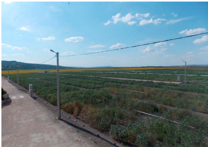
Figure 3. Vertical flow constructed wetland at Orhei's wastewater treatment plant in Moldova, treating municipal wastewater from 20,000 inhabitants [41]. (Courtesy: Iridra Srl— www.iridra.com ).
