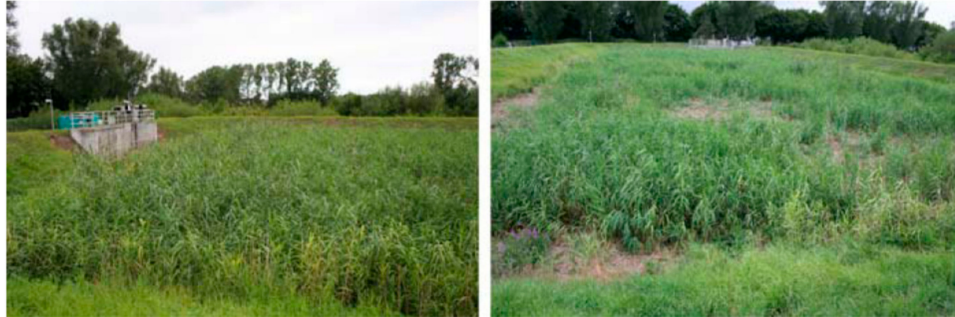
Figure 7. Constructed wetland in Bergheim (Erfurt), Germany for combined sewage overflow (adopted from [79]).
