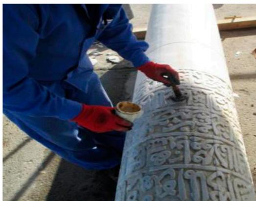
Figure 18. Deep cleaning of a column body.
