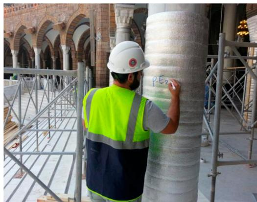
Figure 5. Numbering the column body.
