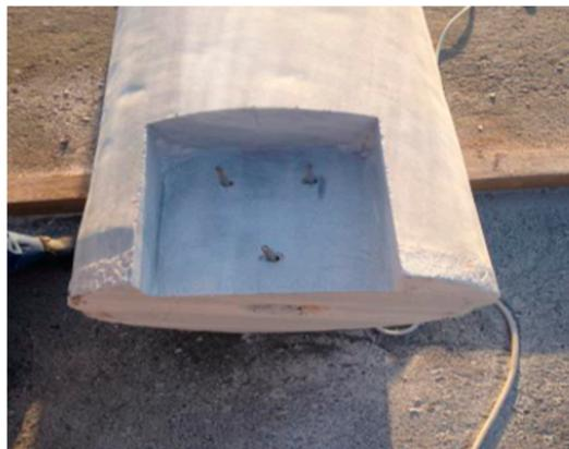
**Figure 23.** Chemical substances and anchors applied.
