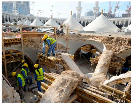
**Figure 12.** Arches stones dismantling.
