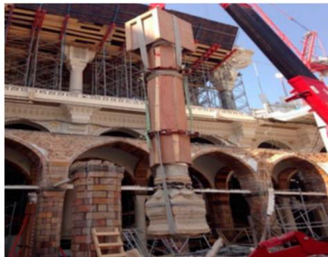
**Figure 8.** Column dismantling.
