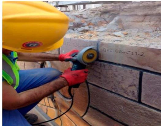
**Figure 11.** Facade stones dismantling.
