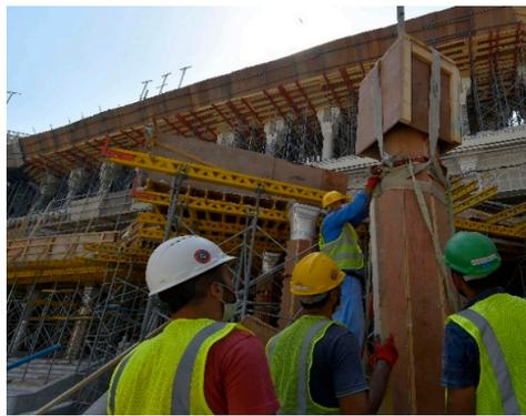
**Figure 7.** Protecting and packing the column.
