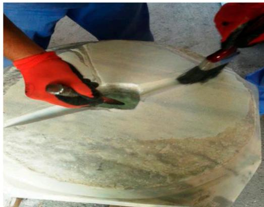
Figure 17. Surface cleaning of a column base.
