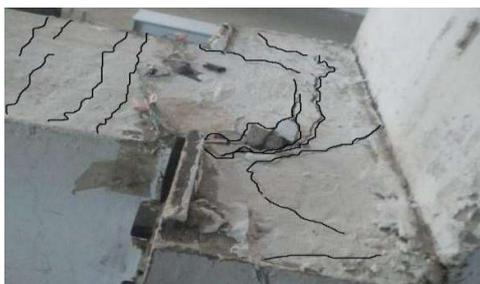
(a) Field photo of cracks on top of beam
