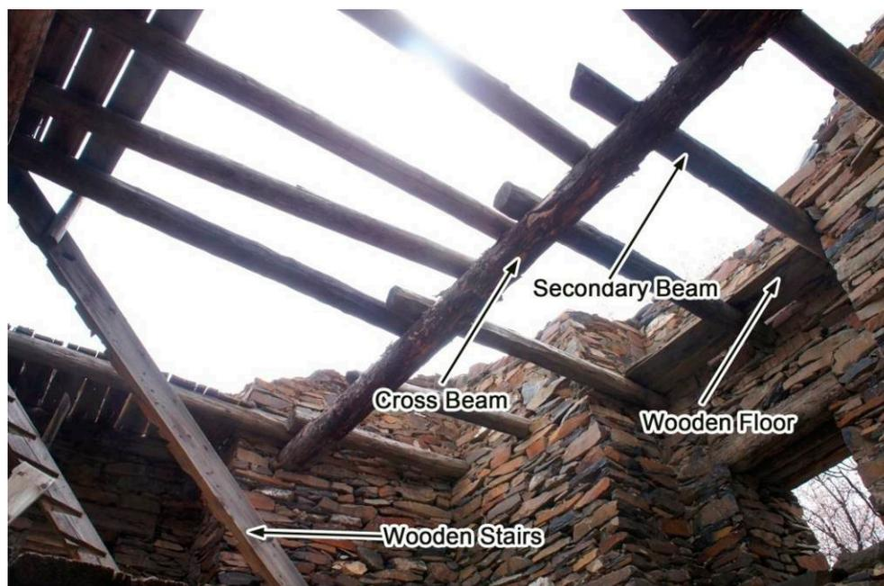
**Figure 11.** Residual wooden beam, plank, and wooden staircase inside watchtower No. 7.
