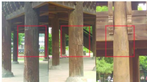
**Figure 12.** Traces of renovation of the exterior columns on the 1st floor. (all figures source: author).
