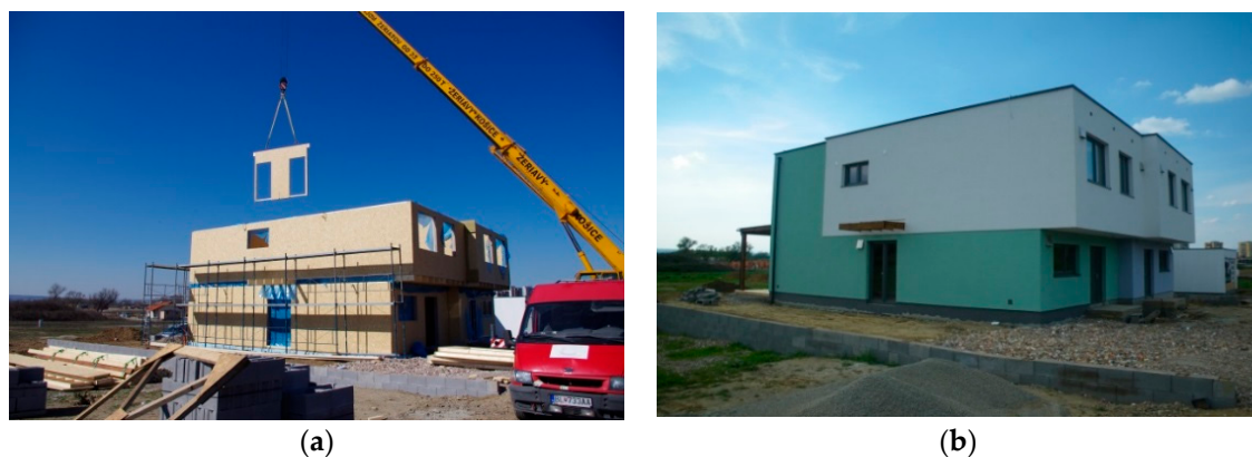
Figure 7. An example of a panel construction (a) Construction process; (b) Panel construction [64].
