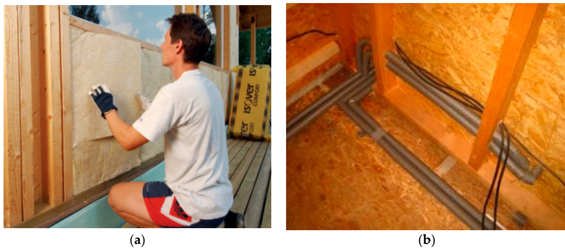
Figure 5. Construction process of details a column construction system (a) Inserting thermal insulation for walls (b) Performing the installation of wiring in the walls [62].
