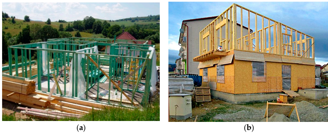
Figure 4. An example of a column construction system (a) Construction process—1st floor (b) Construction process—2nd floor [62].
