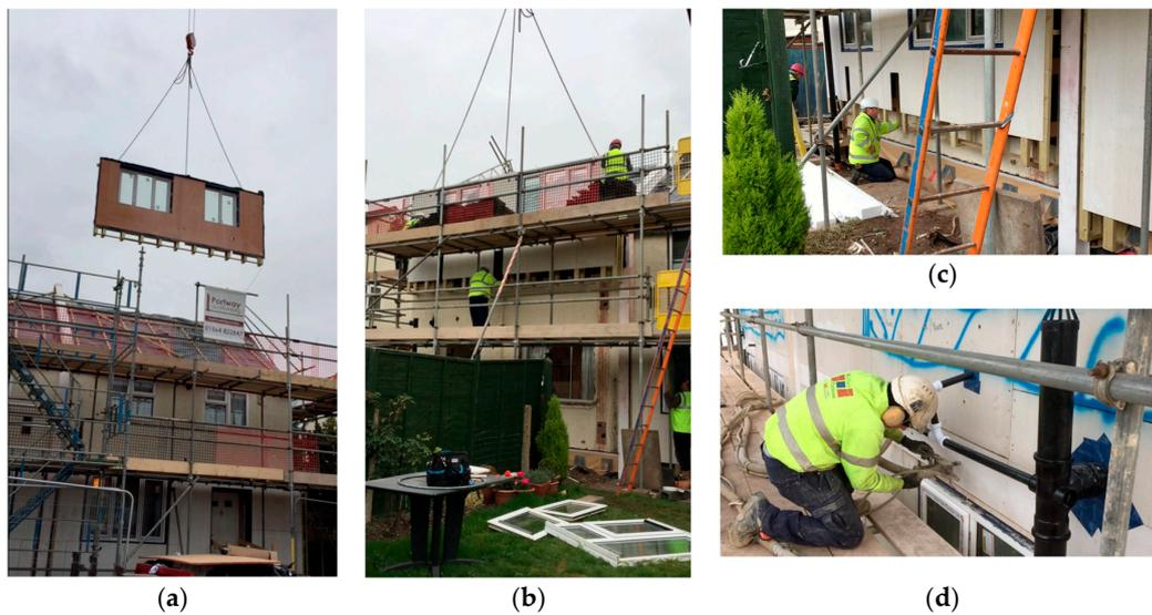
**Figure 3.** Installation of the retrofit thermal envelope: (a–c)—stages of installation of external prefabricated envelope panels; (d) injection of thermal insulation into the installed external panels.
