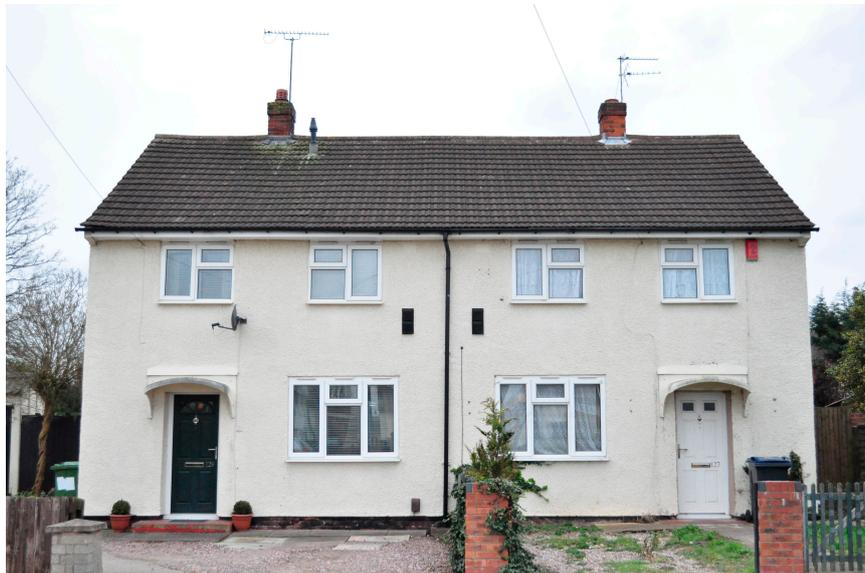
**Figure 1.** Two Wimpey no-fines semi-detached houses before retrofit.
