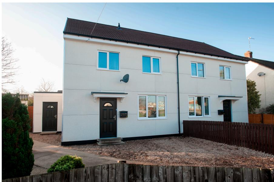
**Figure 4.** Completed retrofit of Wimpey no-fines houses.
