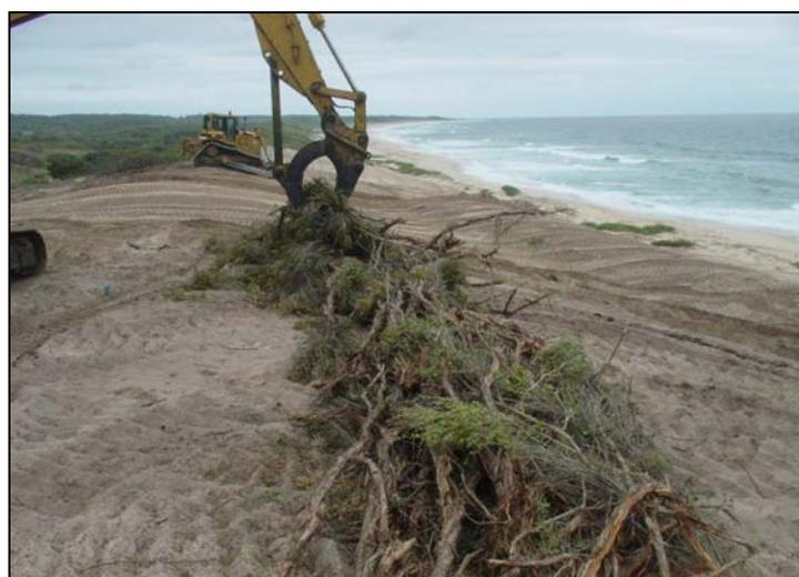
At Magenta, the coastal tea-tree cleared for the golf course was formed into two loosely packed porous windrows along approximately 1.2 km of the re-shaped outer dune. The windrows were placed
