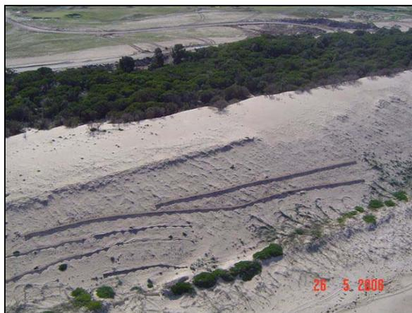
The 200 g/m<sup>2</sup> jute fabric with 40 percent porosity was chosen to capture sand both in front and behind the fence. To minimise blow outs forming, the jute was overlapped in a triangular shape with no sharp defining edge at the ends of each fence. These fences assisted in retaining sand volume in the reconstructed dunes.
