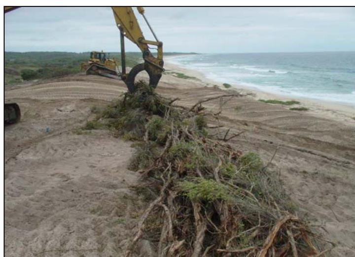
At Magenta, the coastal tea-tree cleared for the golf course was formed into two loosely packed porous windrows along approximately 1.2 km of the re-shaped outer dune. The windrows were placed
