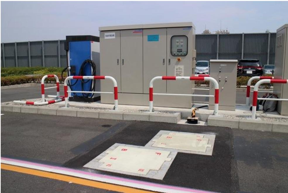
**Figure 5.** Transmit equipment of 85 kHz band 44 kW wireless rapid charging system.
