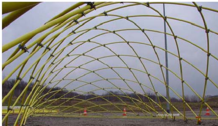
Figure 2. Single layer gridshell constructed of GFRP poles [9].
