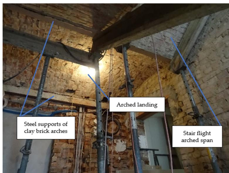
**Figure 5.** View of the researched masonry staircase.
