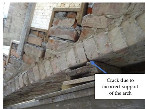
**Figure 7.** Section of the staircase with visible crack of the arch caused by improper renovation and deterioration of masonry joints.
