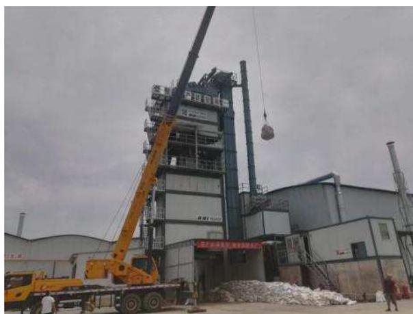
**Figure 8.** Hoisting the snow-melting salt into the mixing plant.
