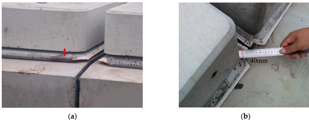
**Figure 2.** The gap between filling layer and track slab (a) vertical direction, (b) horizontal direction.
