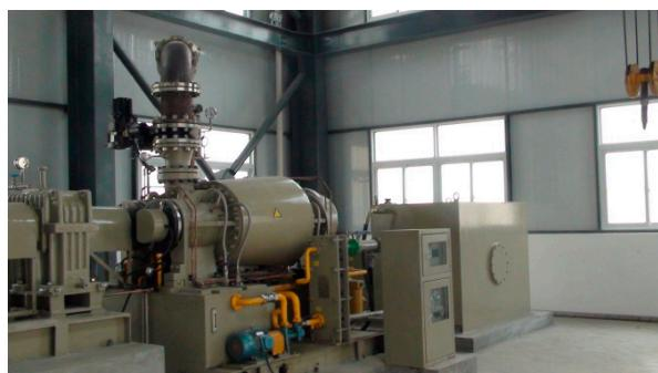
**Figure 1.** The second screw expander generating unit in YangBaJing geothermal power plant.
