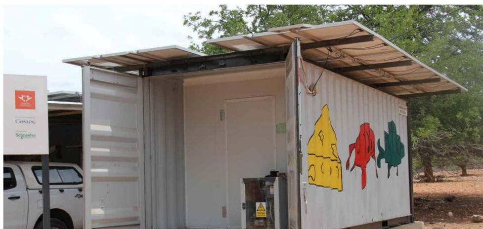
**Figure 1.** Gwakwani village PV-powered cold storage.
