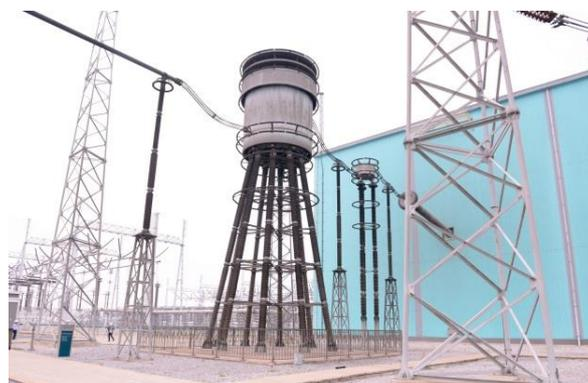
**Figure 1.** Pole bus smoothing reactor of the Jiaodong  $\pm 660$  kV converter substation.
