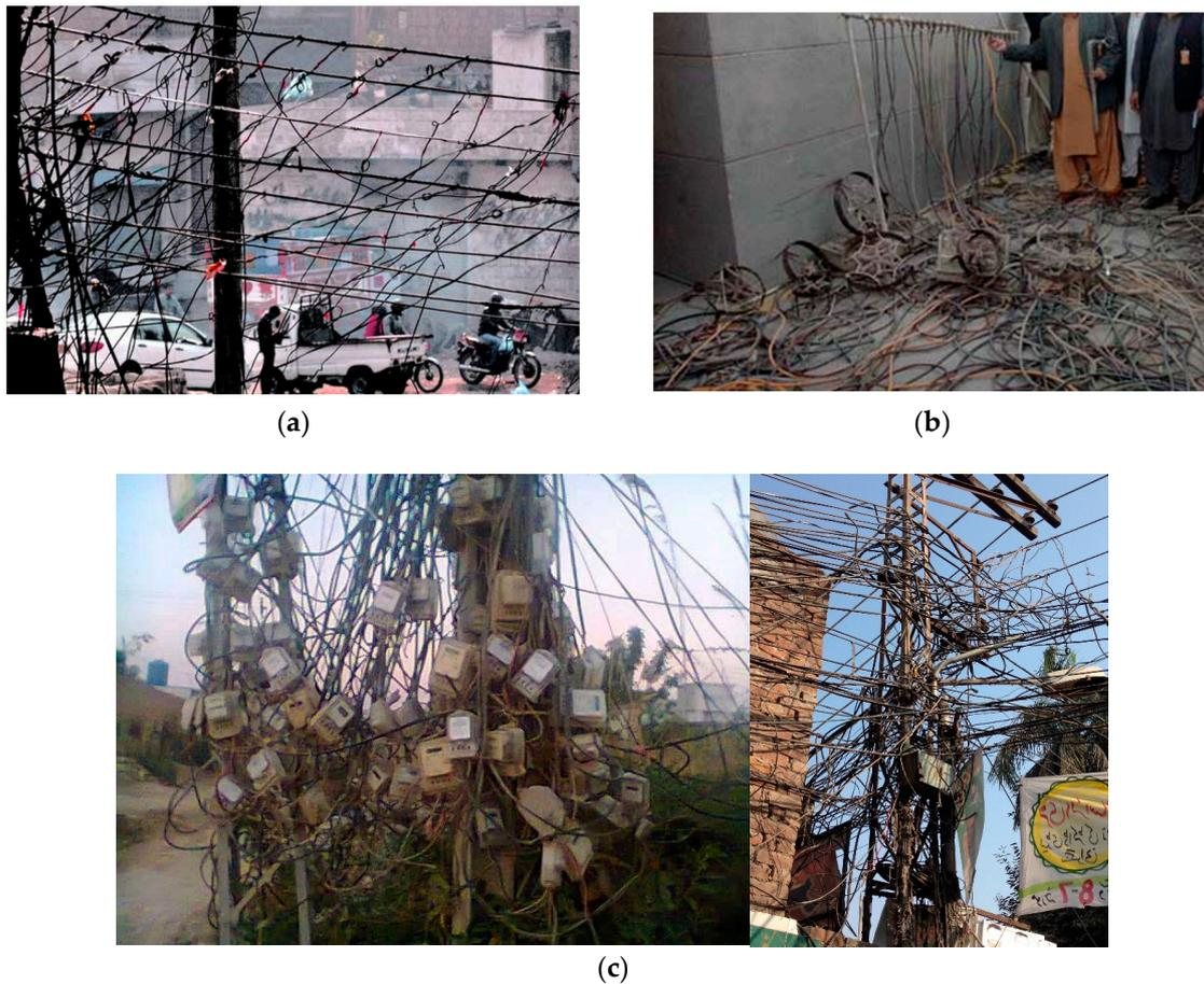
**Figure 6.** (a) Illegal electricity connections—the use of hook (kundas) on main electricity supply lines in Karachi, Pakistan, bypassing electric meters [39]; (b) Illegal gas connections in Lahore, Pakistan, bypassing gas meters [40]; (c) Conditions of electricity meters on electric poles (impossible to isolate energy consumption by consumer). Photo credit: unknown.
