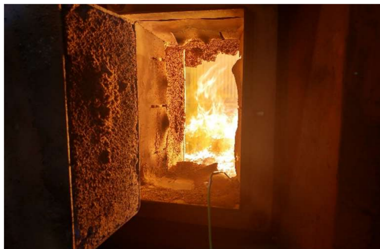
Figure 4. The middle part of grate—view from the middle inspection door of the boiler.
