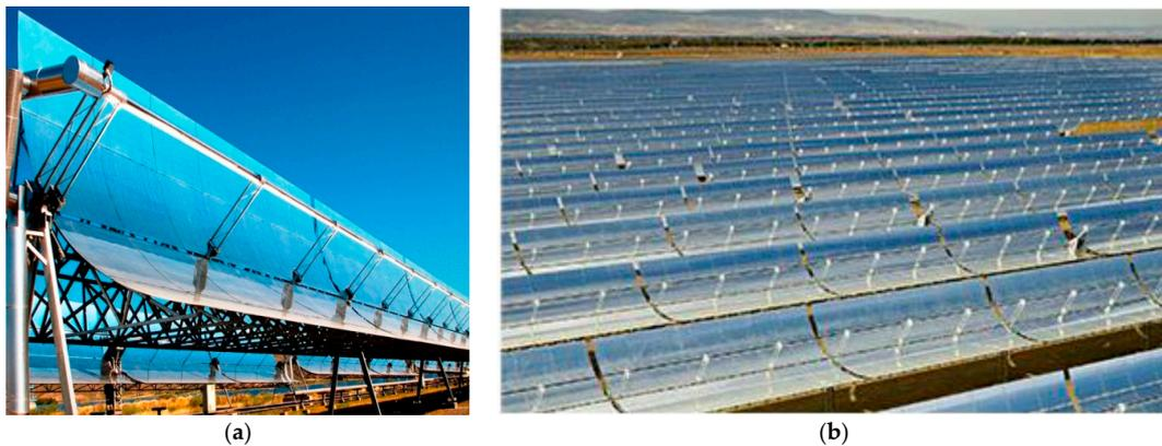
**Figure 3.** Concentrated Solar Power Technologies: (a) parabolic cylindrical collector; and (b) parabolic trough solar power plant—ANDALUSIA AND SOL I—ANDASOL I (50 MW, Granada, Spain).
