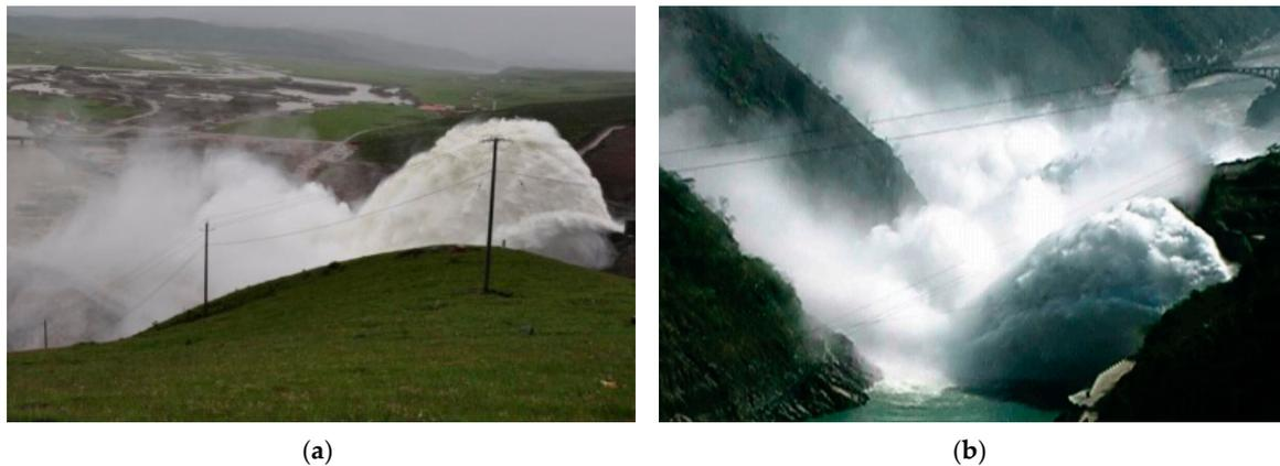
**Figure 1.** Flood discharge atomization caused by trajectory energy dissipation. (a) Nazixia Hydropower Station and (b) Dongjiang Hydropower Station.
