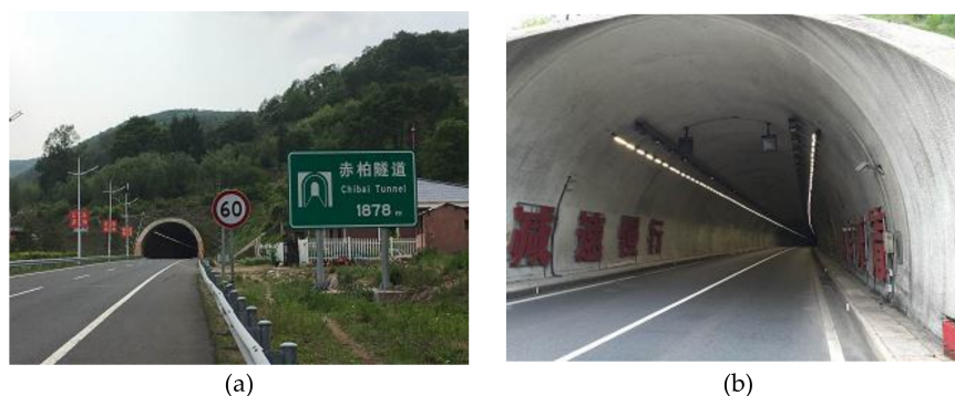
Figure 1. Chibai Tunnel, (a) Entrance to the tunnel; (b) LED luminaries installed in the tunnel.
