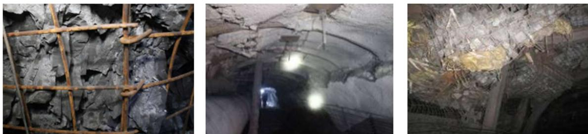
**Figure 1.** Failure phenomenon of broken surrounding rock in deep coal mine roadway.
