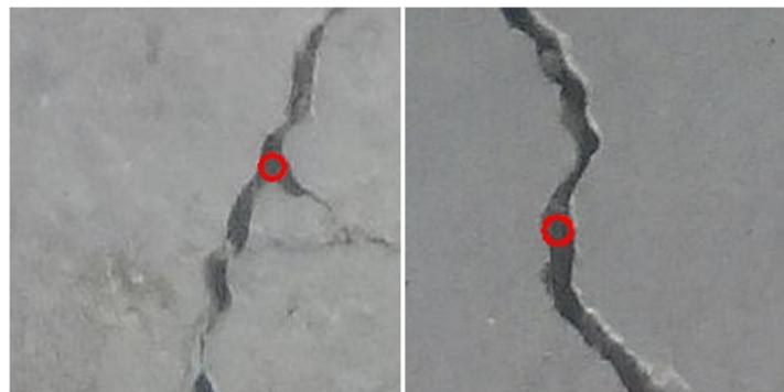
Figure 9. Visual annotation of maximum crack width.
