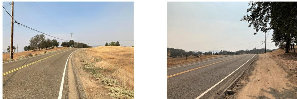
**Figure 4.** Example rural intersection from the point of view of vehicles traveling north–south through the intersection. Note the lack of visibility across the intersection.
