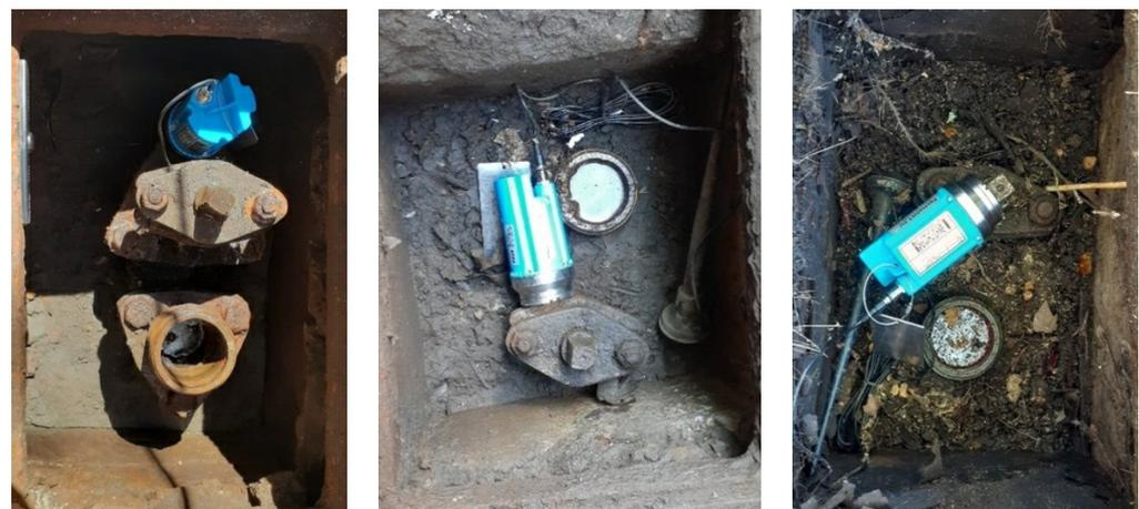
**Figure 2.** HWM PermaNET SU loggers deployed on hydrant control valves in different locations.
