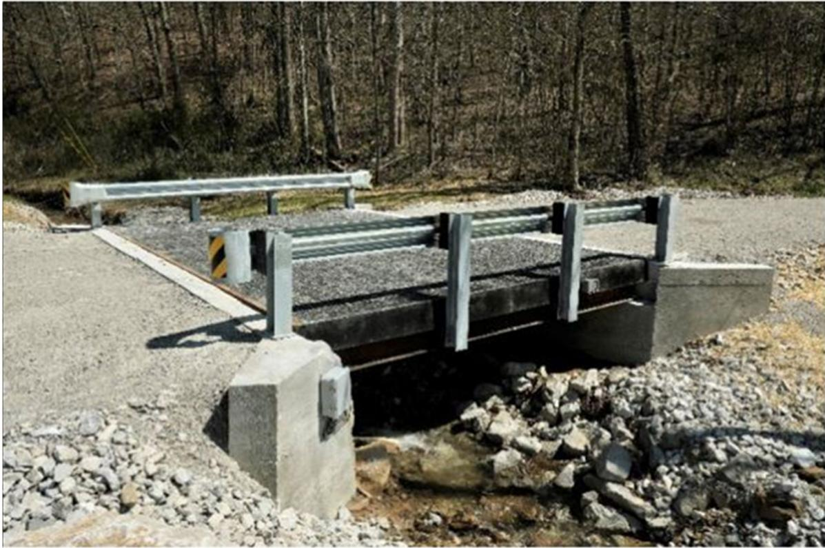
**Figure 3.** Photograph of the installed fiber-reinforced polymer composite bridge supported by steel girders.
