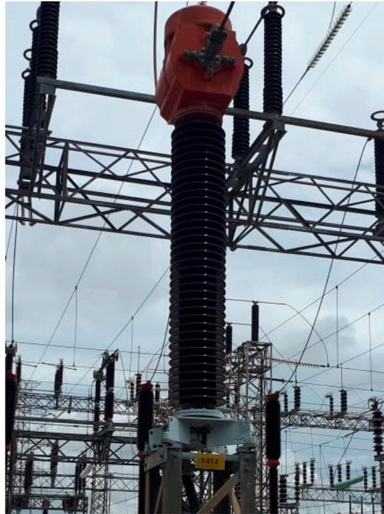
**Figure 14.** The 230 kV Current Transformer evaluated in the field application tests.
