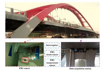
Figure 2. Deployment of FBG-based SHM system.
