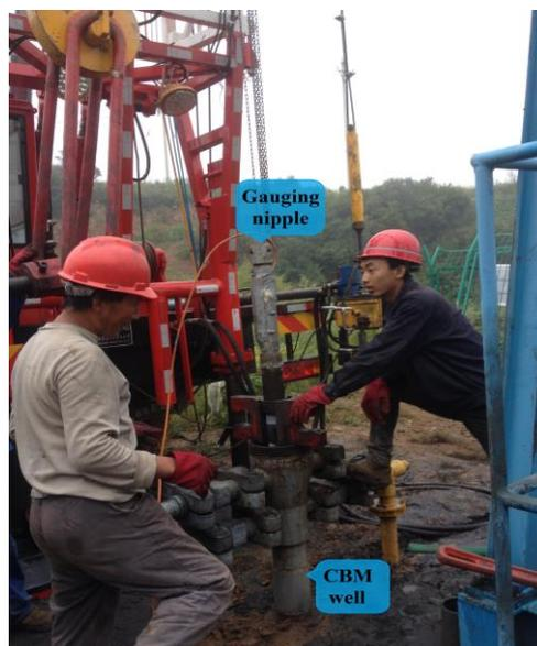
**Figure 10.** Field of the gauging nipple entering the well.
