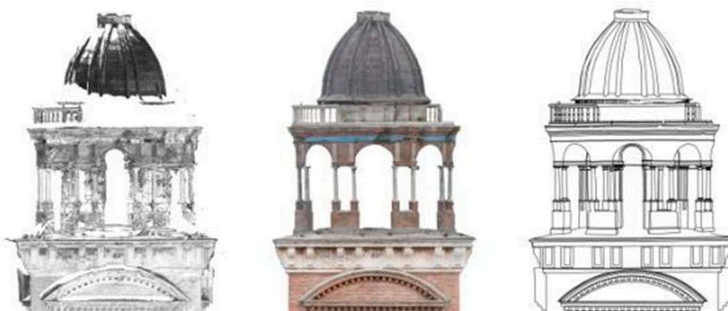
**Figure 9.** Comparison between the Santa Barbara bell tower's top laser scanner data and the respective surface orthophoto elaborated from the photogrammetric 3D model.
