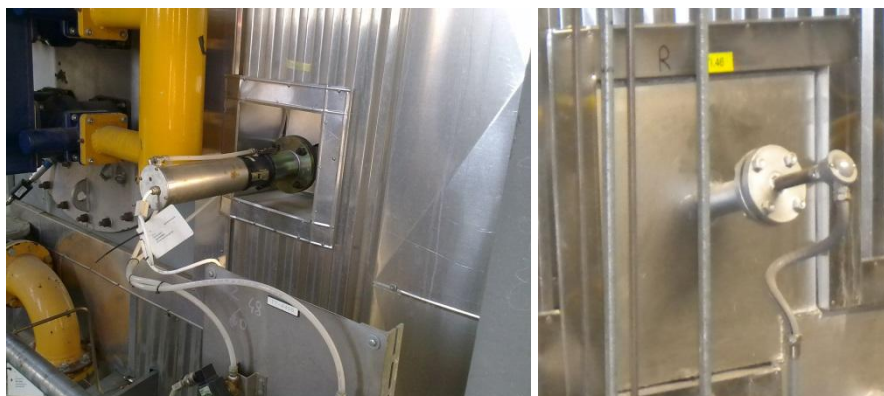
Figure 4. External views of an infrared radiation (IR) pyrometer on the left and of a bare thermocouple on the right, both installed on a WTE boiler.
