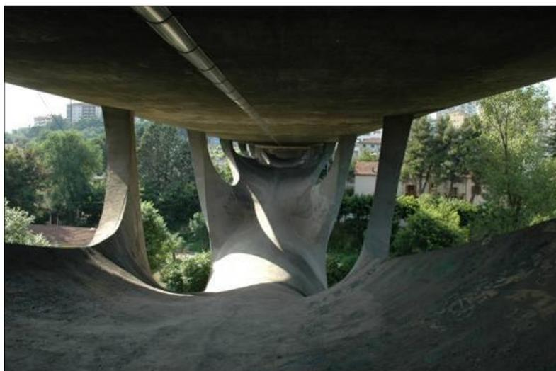
At present, the bridge, constituted by reinforced concrete, shows related aging problems and causes worries related to the recent growth of the traffic load. A monitoring plan of this important structure having a direct impact on the lower railway line is necessary.
