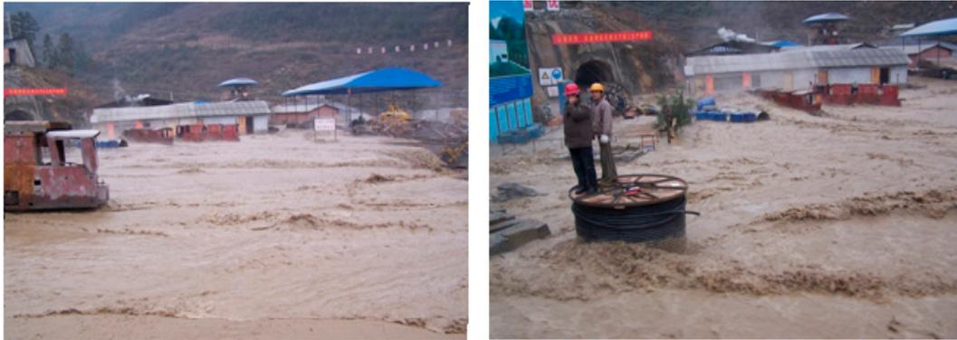
**Figure 3.** An accident due to water inrush in the Malujing tunnel of Yiwan railway.
