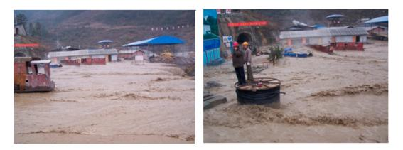
Figure 3. An accident due to water inrush in the Malujing tunnel of Yiwan railway.
