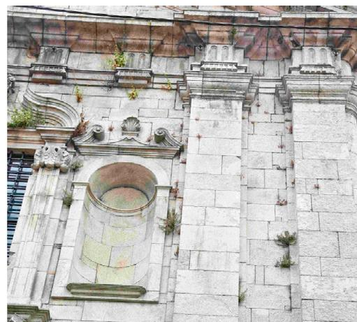
**Figure 29.** Identification of the various pathologies on the north façade of Vitória Church, Porto.
