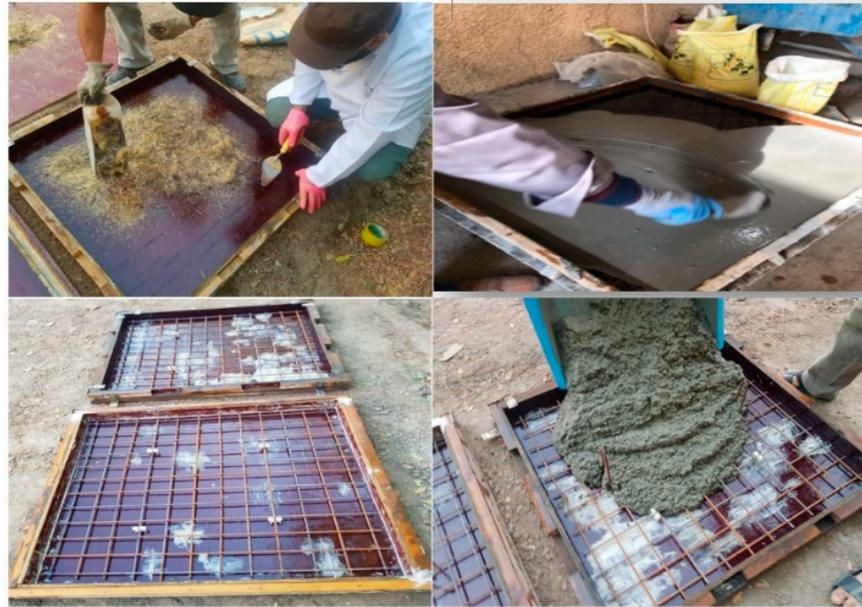
**Figure 3.** The casting of SIFCON and NSC slabs.
