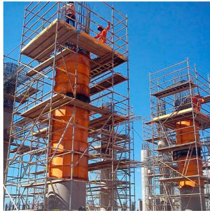
**Figure 1.** Work on circular columns using formwork and scaffolding [5].
