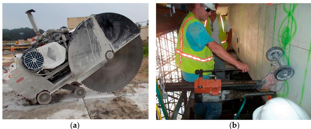
**Figure 2.** (a) A diesel-operated slab saw. (b) The drilling operation conducted on the side of the beam.
