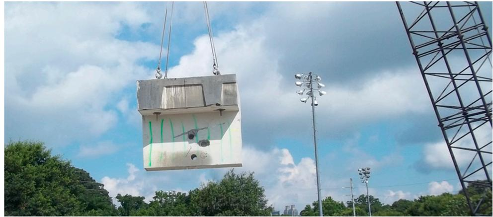
**Figure 3.** Lifting of a cut segment of the PT beam.
