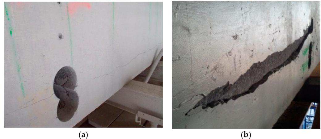
**Figure 9.** Horizontal cracking (a) and spalling of concrete (b) on the side of the beams as the result of drilling and cutting tendons.
