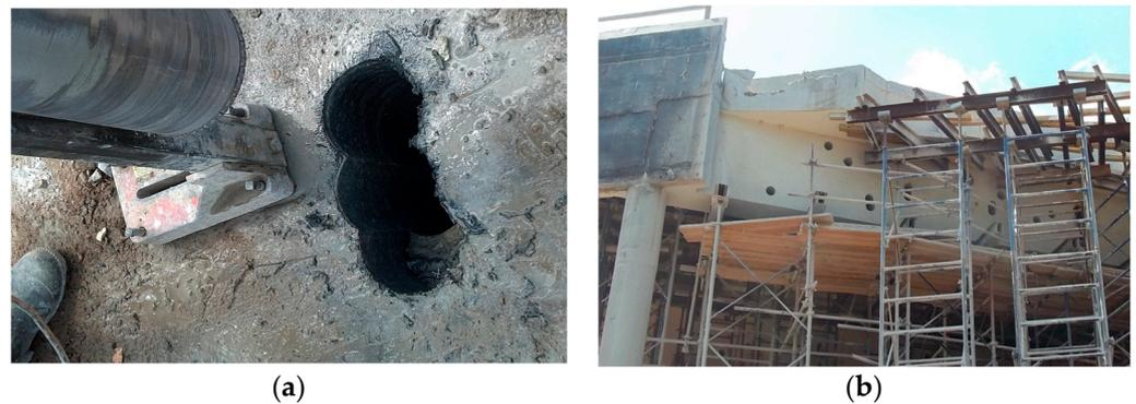
**Figure 6.** (a) The drill and holes on top. (b) Side view of one of the beams showing the considerable number of drillings required to locate and cut the PT ducts.
