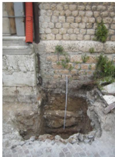
**Figure 17.** Photo of the inspection Pit, IP, near the foundation of the belfry, taken by Fine Art Authority.
