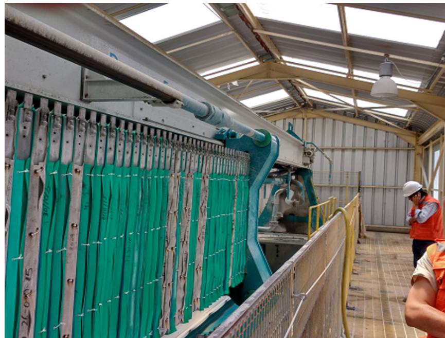
Figure 40. Tambo de Oro Tailings Vertical Plate Filter Press [49].
