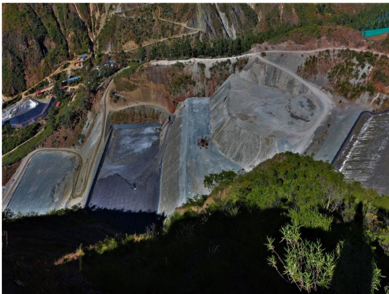
Figure 66. Curaubamba Filtered TSF—Benches and Terraces [38,39].
