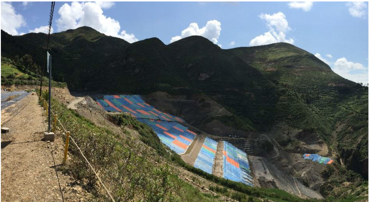
Figure 67. Ramahuayco Filtered TSF—Terraces Overview [40,41].
