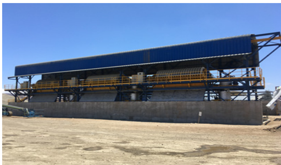
Figure 44. Tambillos Tailings Ceramic Disc Filters [48,66].
