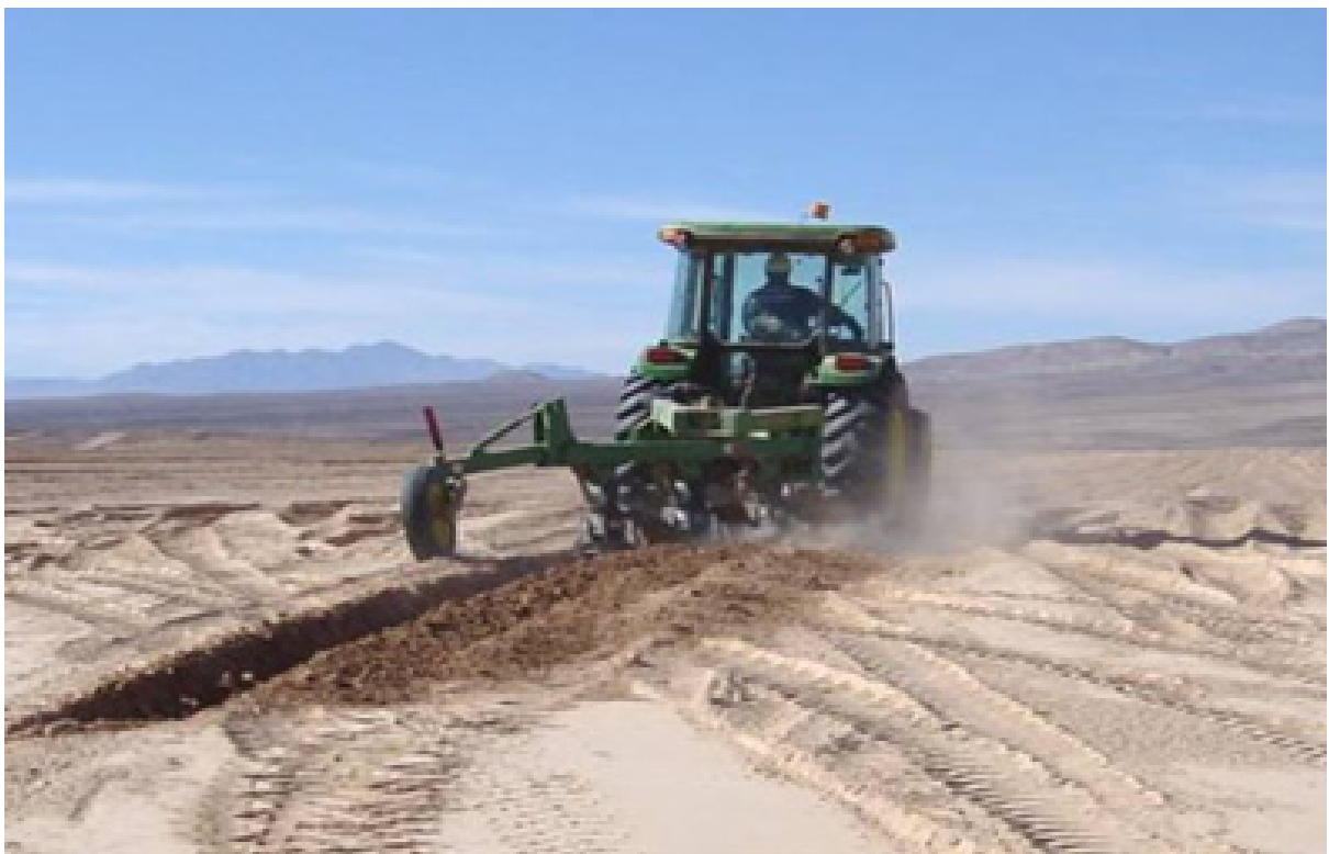
Figure 33. El Peñon Filtered Tailings Storage Facility—Tailings are removed by a disc plow [62,63].
