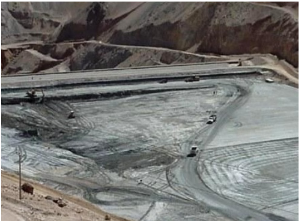
Figure 23. El Indio Filtered TSF Overview—Haul Trucks and Dozers works [53].
