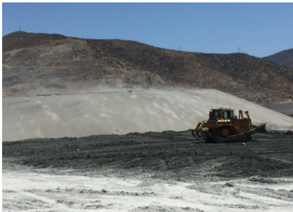
Figure 39. Salares Norte Filtered Tailings Storage Facility—Dozer forming filtered tailings layers [50,64,65].
