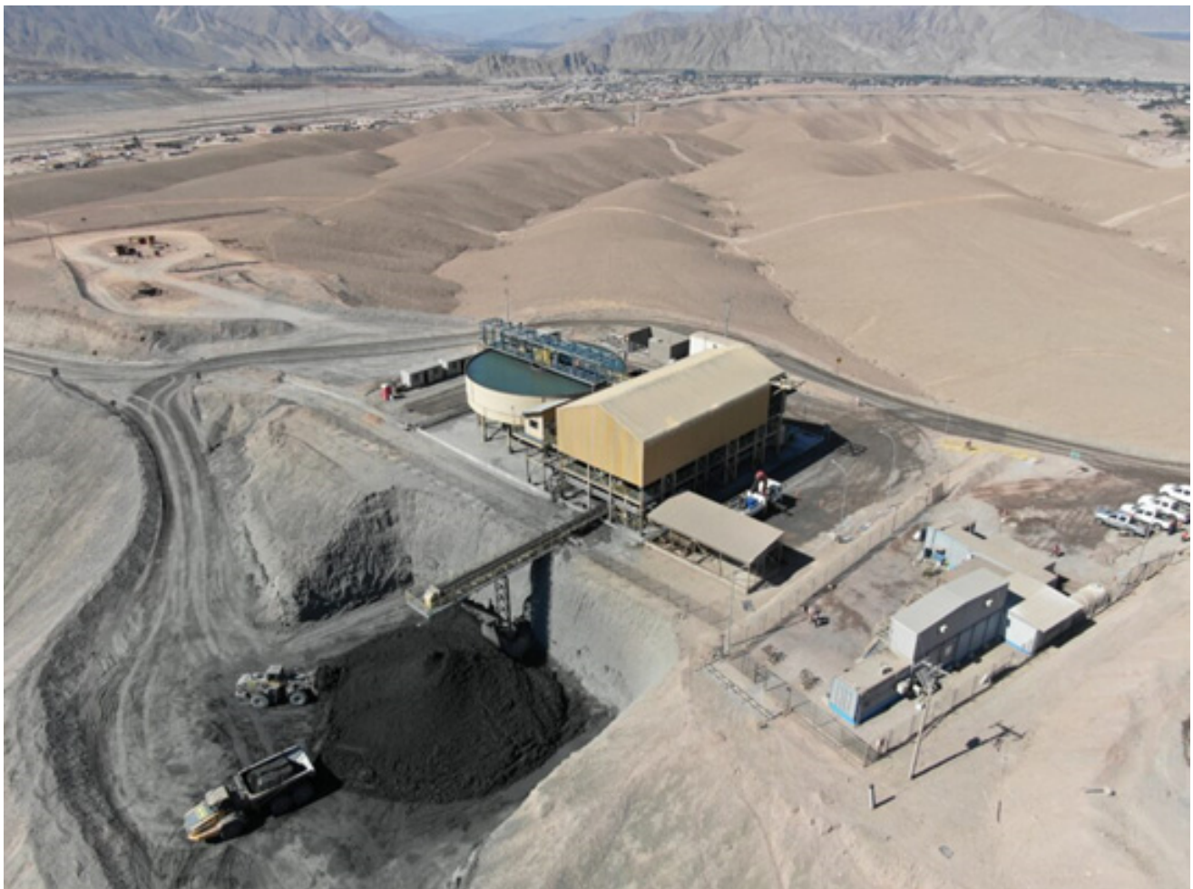
Figure 28. El Gato Creek Filtered Tailings Plant [27,47,61].
