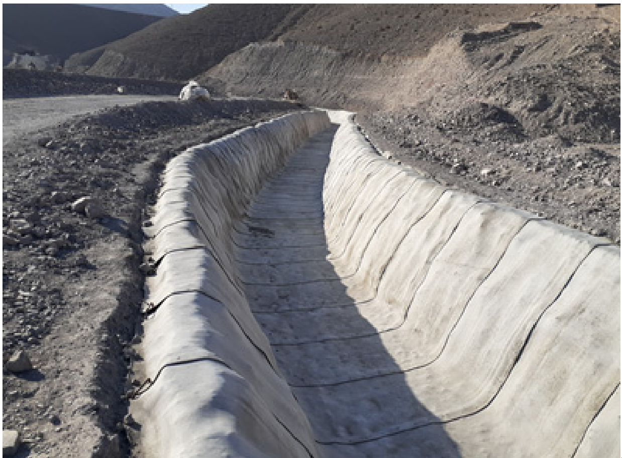
Figure 18. Collection and diversion system for non-contact water-perimeter ditches [27].
