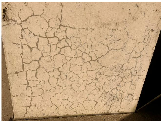
**Figure 1.** Concrete column affected by the alkali-silica reaction (ASR) presenting a map cracking pattern.
